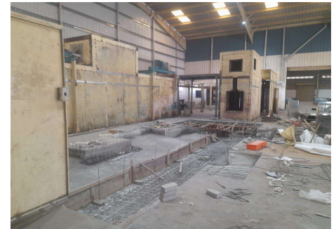
Paint Shop Construction Picture
